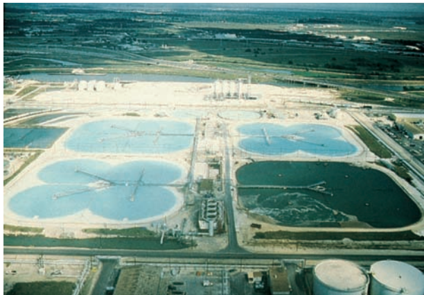
Magnesium hydroxide was precipitated from processed seawater in settling ponds The Dow Chemical Company once operated.
